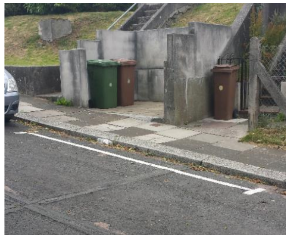
Access protection markings installed at Severn Place (Efford & Lipson) (↑)
