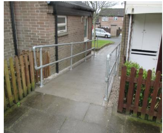
Access ramp installed to assist disabled access at Vermont Gardens (Ham) (↑)
