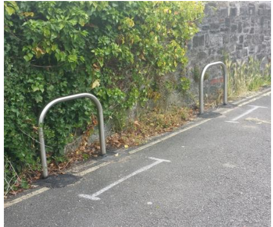
New cycle parking installed at Crownhill Village (Eggbuckland) (↑)
